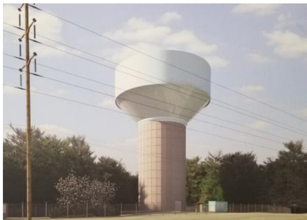
Hickory Hills Water Storage Tower
