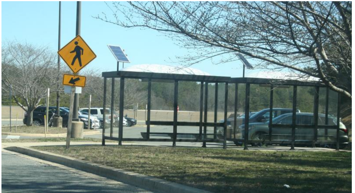
The Park and Ride on Airport Road will have to be suspended and relocated while the road is moved closer to University System of Maryland at Southern Maryland
