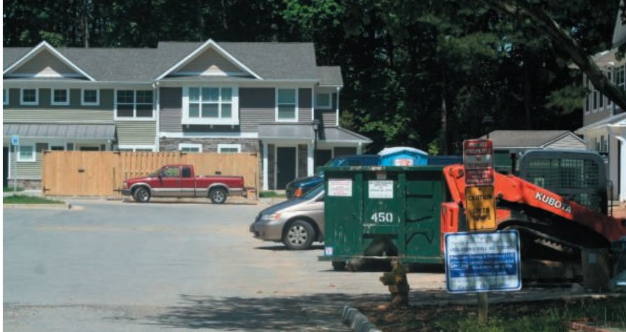
Renovations continue at Lex Wood apartments in Lexington Park
