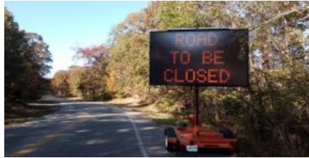
A portion of White Oak Parkway will be closed to replace an aging drainage culvert.
