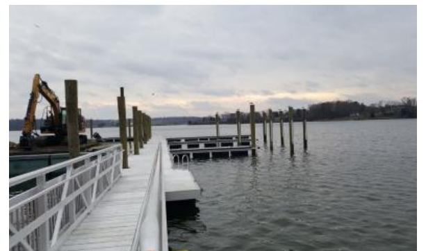
Phase 1 of the Leonardtown Wharf Pier
