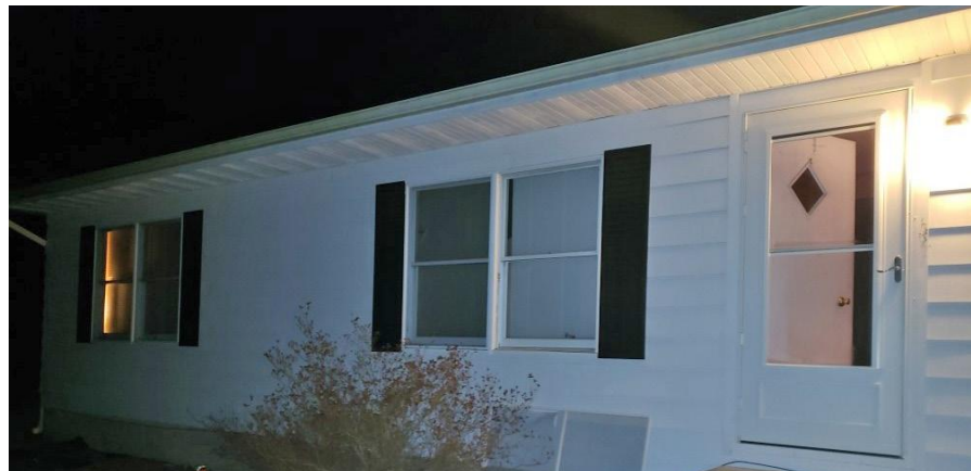
A fire at a Wheatley Avenue residence has been deemed arson.
