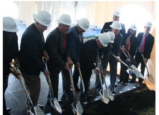
Leaders break ground on the new CBOC in Charlotte Hall
