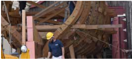
COMMUNITY 12 Work continues on construction of the new Maryland Dove.
