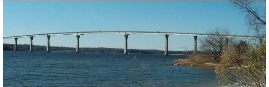
Gov. Thomas Johnson Bridge
