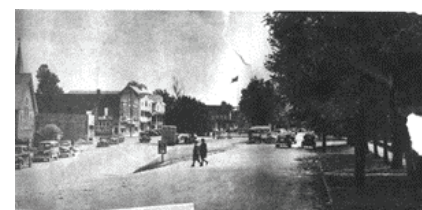
Leonardtown in 1949 looking west along Washington St. Note the dirt road.
