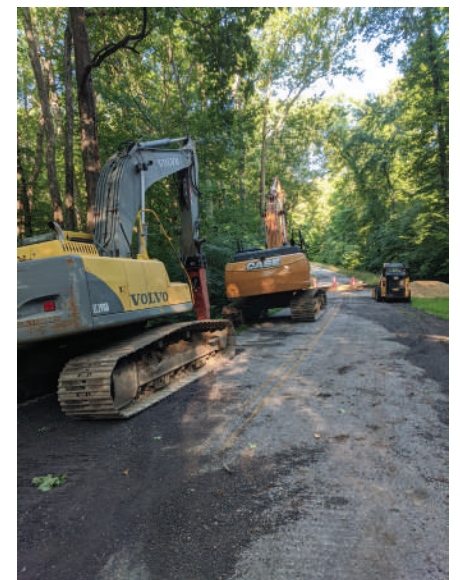
Construction equipment set up near Manor Bridge Road
