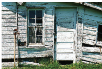
The outside water faucet - still in place today.
