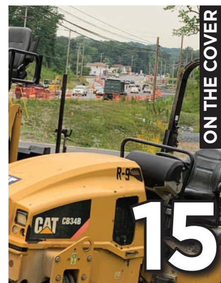
Town officials hope for a swift end to Route 5 project.
