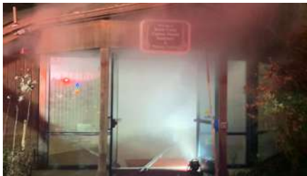
LOCAL 5 Nature center damaged in fire
