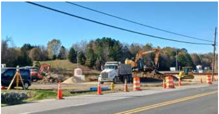
LOCAL 8 Hollywood Square Construction Begins
