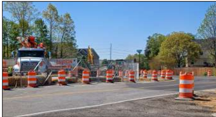
LOCAL 6 Buck Hewitt Road project continues
