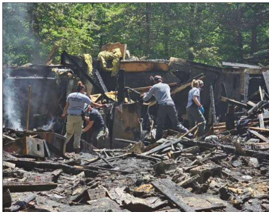
The aftermath of the fire on Deerwood Park Drive
