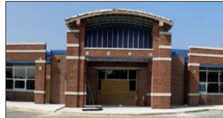
LOCAL 8 School renovations underway
