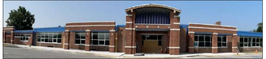
The new façade at Mechanicsville Elementary School
