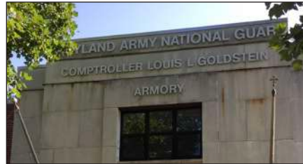
LOCAL 6 Prince Frederick Armory demolished
