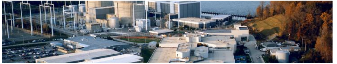
LOCAL 7 Drill planned for Calvert Cliffs emergency operations center.
