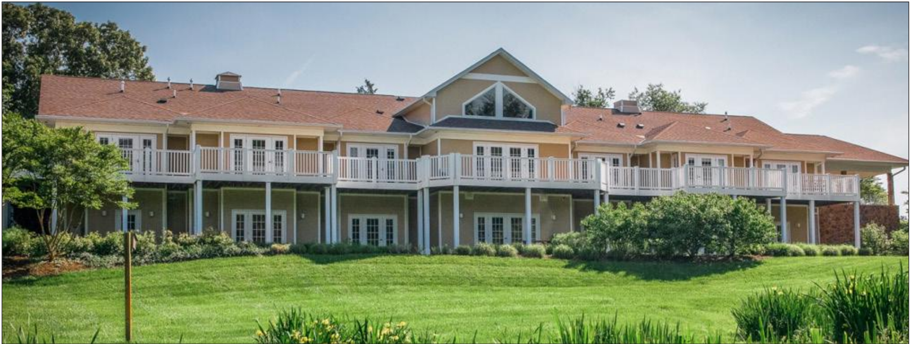
Back of Burnett Calvert Hospice House showing the deck and the backs of the hospice units.
