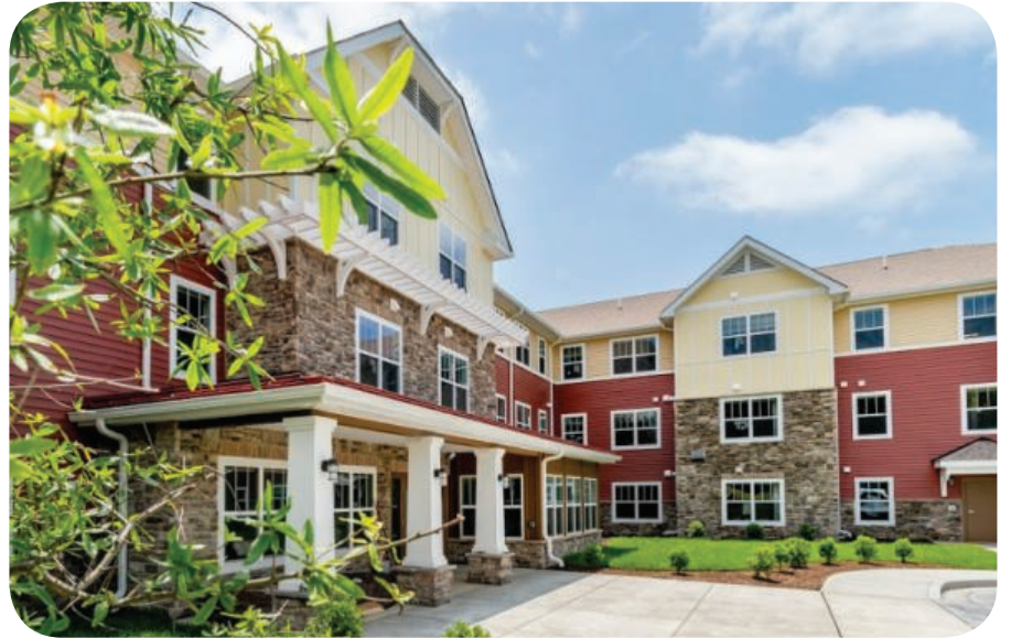
Southern Pines II senior housing complex
