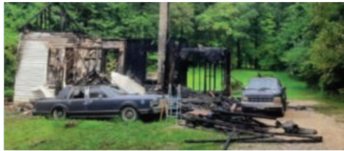
COMMUNITY 11 Fatal house fire probed
