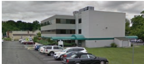
LOCAL 6 The County Services Plaza will be demolished.
