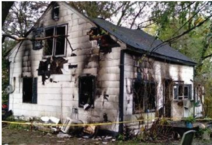
Charred remains of the Harrod home in Lusby.
