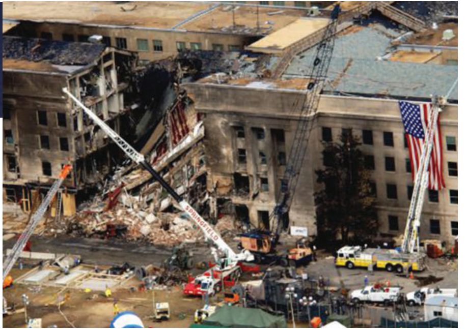
Aerial view of the damage at the Pentagon
