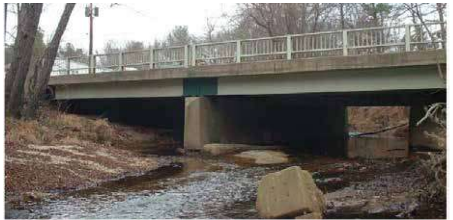
The Route 5 bridge in Great Mills over the St. Mary's River
