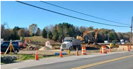
LOCAL 8 Hollywood Square Construction Begins
