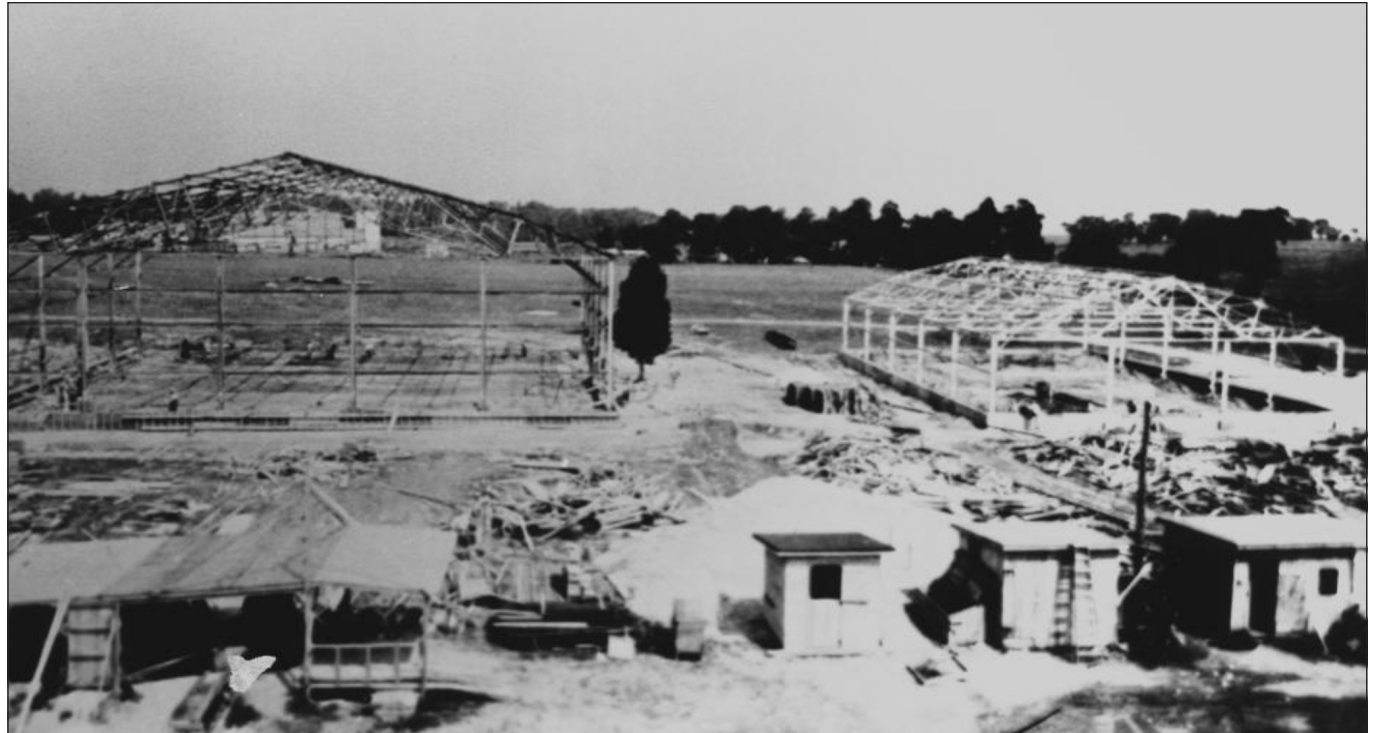
Construction of Naval Air Station Patuxent River began April 4, 1942.
