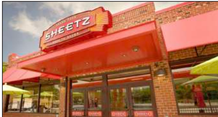
LOCAL 5 Charlotte Hall Sheetz approved
