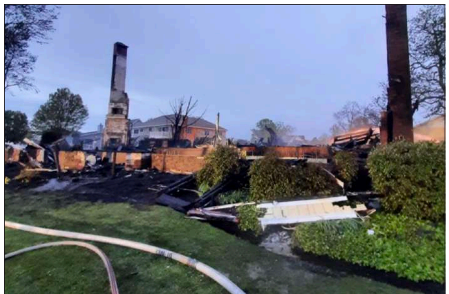
The aftermath of the fires at Champion Used Auto Parts (top) and a Tall Timbers home (bottom). Photos courtesy of Maryland State Fire Marshal.
