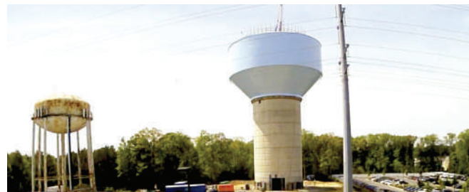
LOCAL 7 New water tower takes shape in Hickory Hills.
