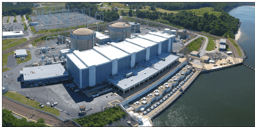
Calvert Cliffs Nuclear Power Plant
