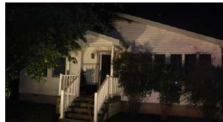
LOCAL 6 Fire damages Lusby home
