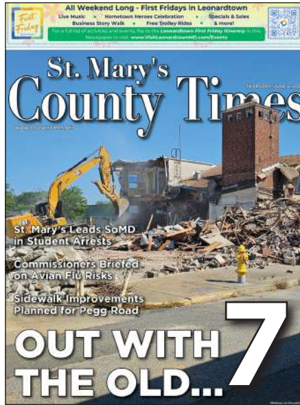
ON THE COVER 7 Demolition of Tulagi Place underway
