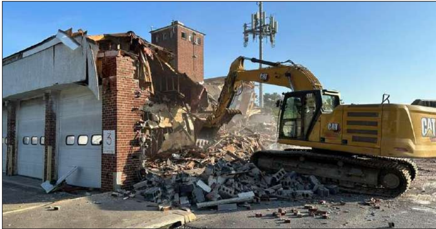
Demolition of the vacant firehouse on South Coral Drive
