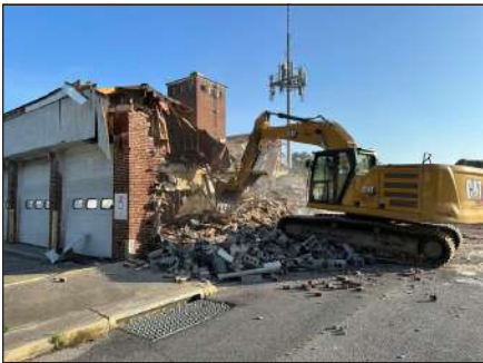
Demolition of the old firehouse on Great Mills Road
