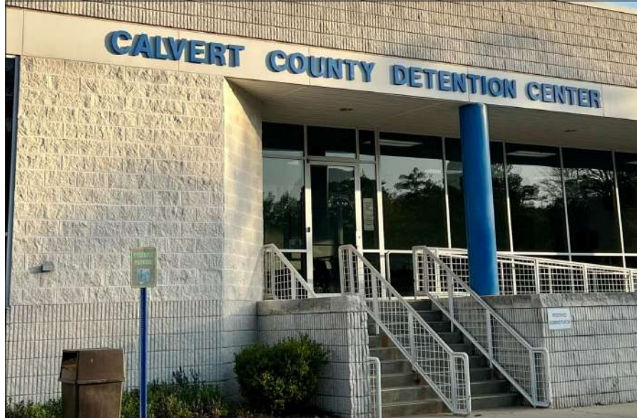
Calvert County Detention Center
