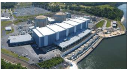
LOCAL 5 Calvert Cliffs wraps up refueling outage
